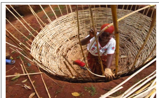
The picture shows a lady weaving a water harvesting tank using bamboo
